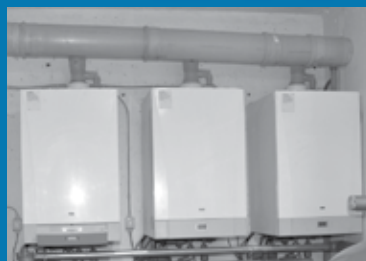
Central Baxi high efficiency boiler plant
