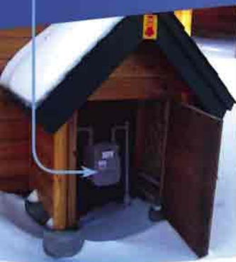
■ Meter with snow shelter
